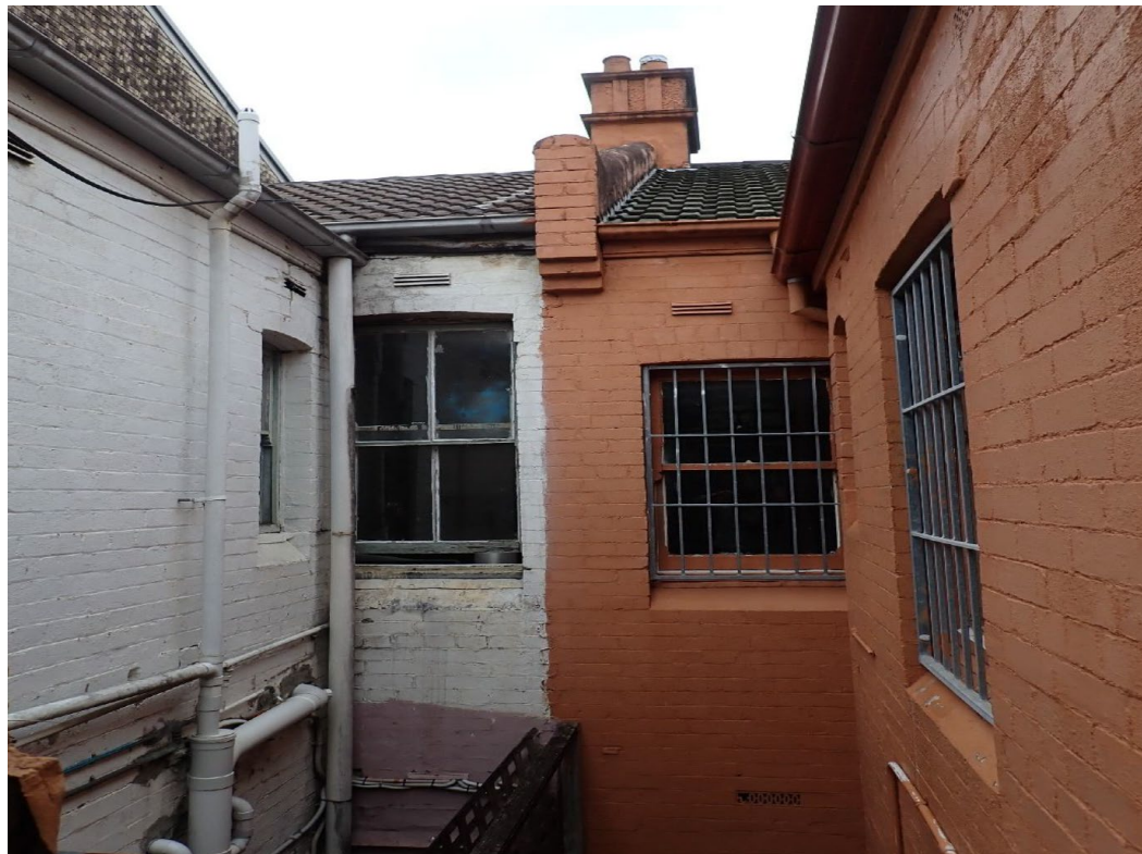
View from first floor external stair showing party wall and neighbouring development facing east
