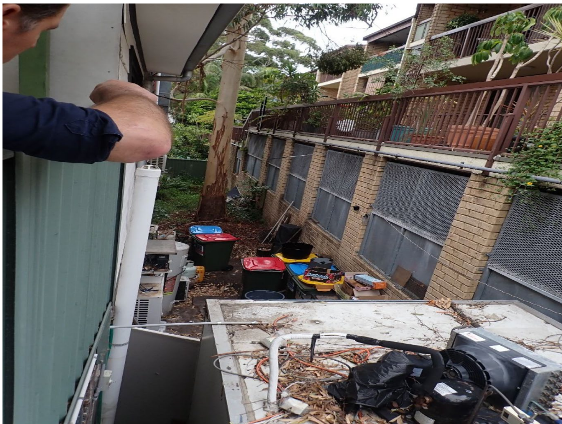
View from first floor external area showing private lane including cold room and tree facing south
